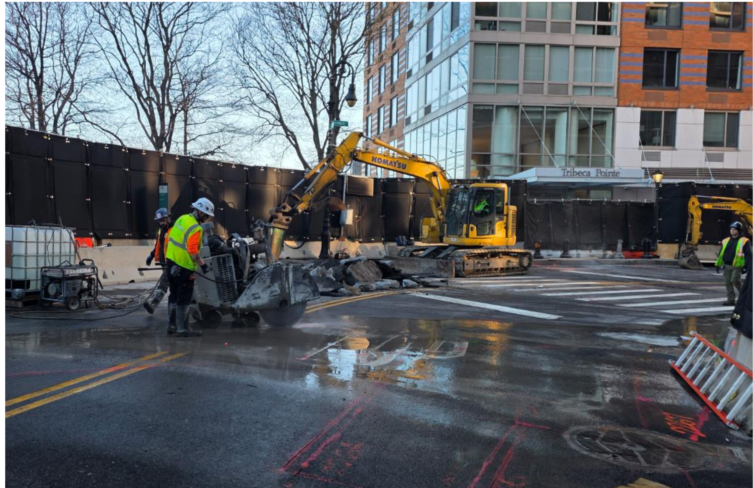
Surface demolition and salvage
