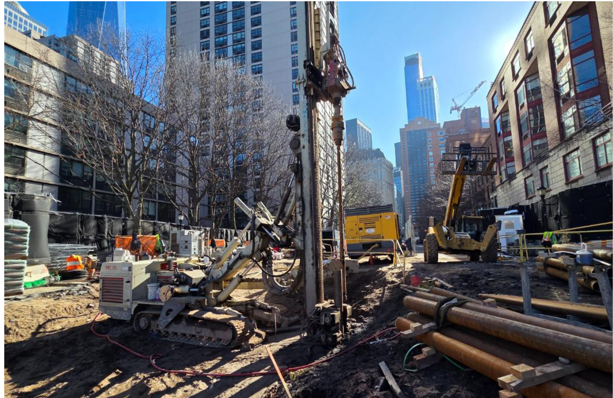
Pile drilling for the Tide Gate installation
