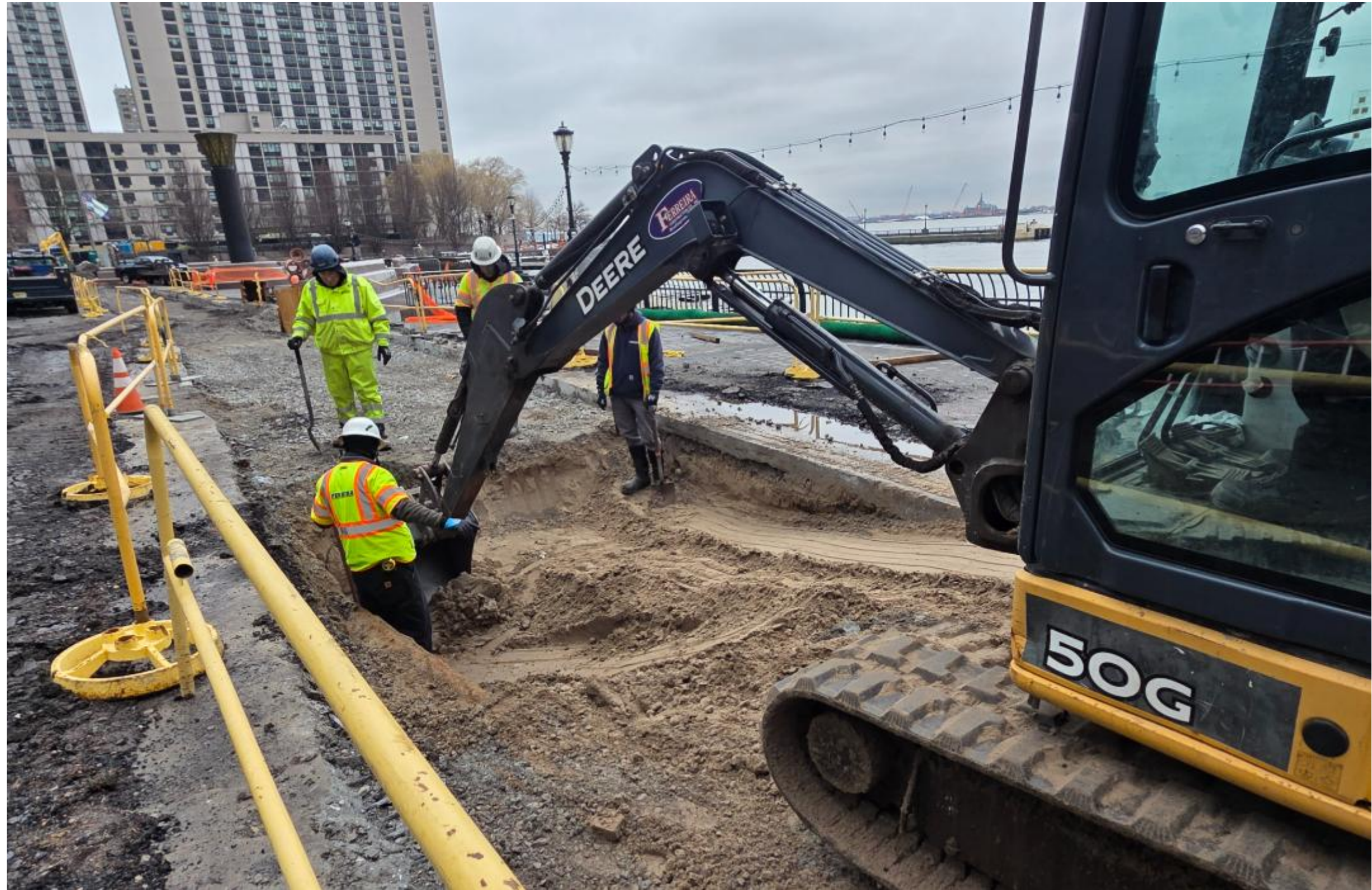
Excavation of ECS trench
