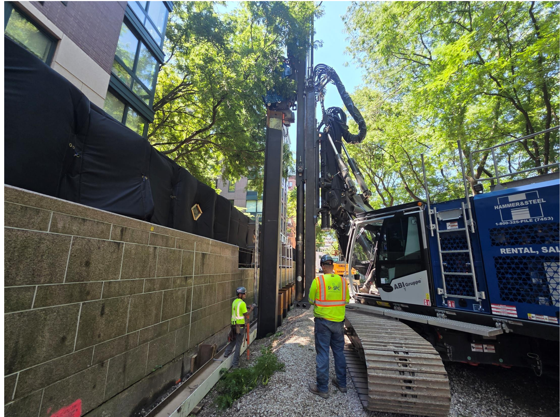
Sheet pile installation along Riverwatch
