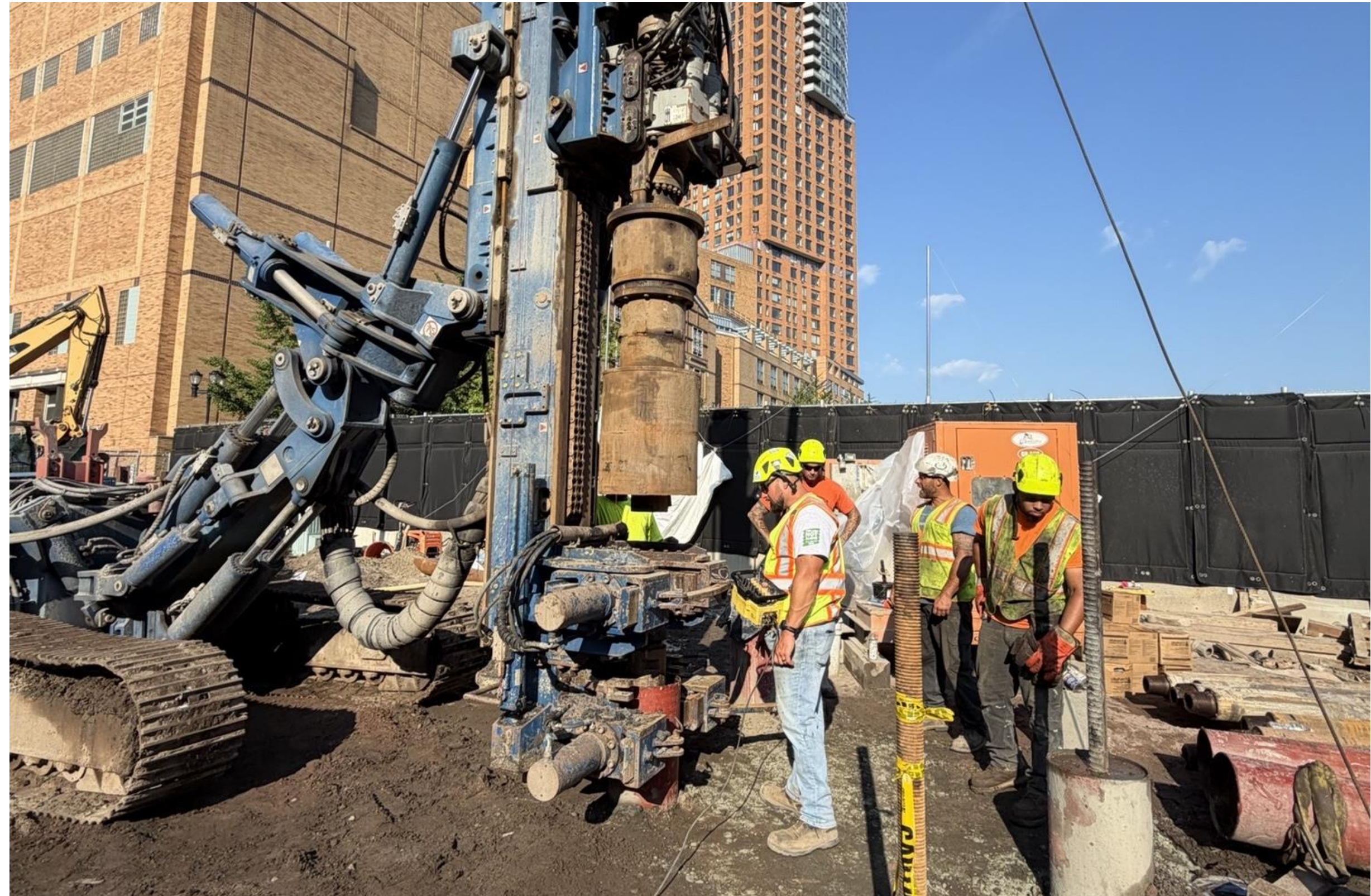
Pile Installation along Route 9A
