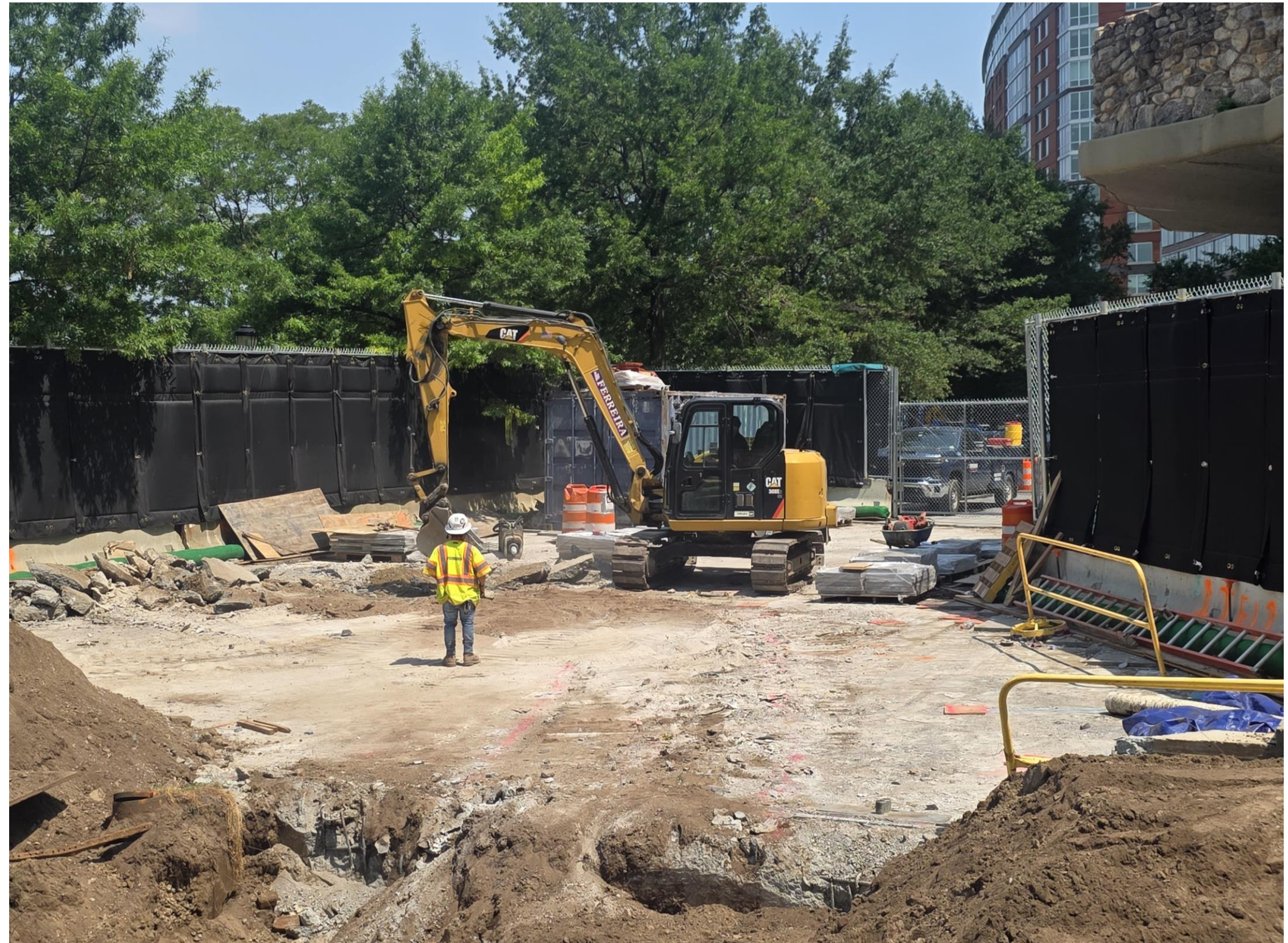
Surface demolition and salvage underway
