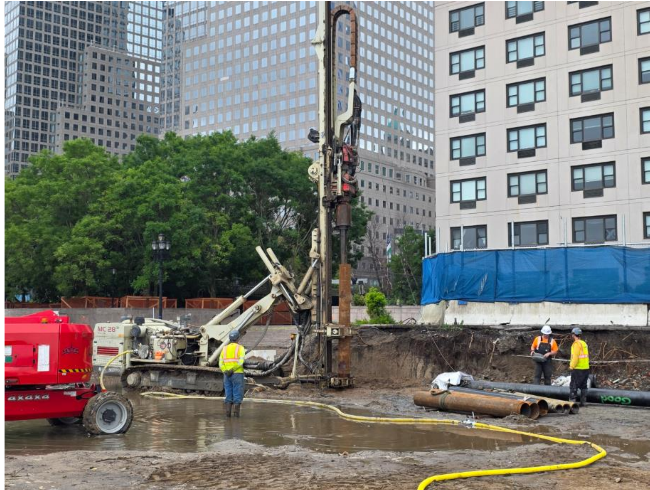
Pile Installation at Gateway Plaza
