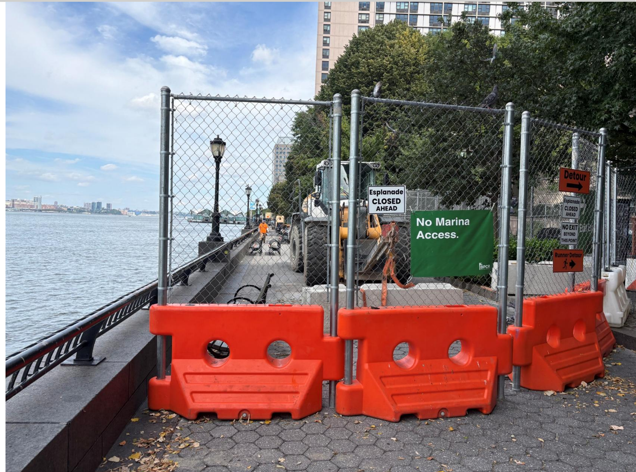
Esplanade closure at Albany Street
