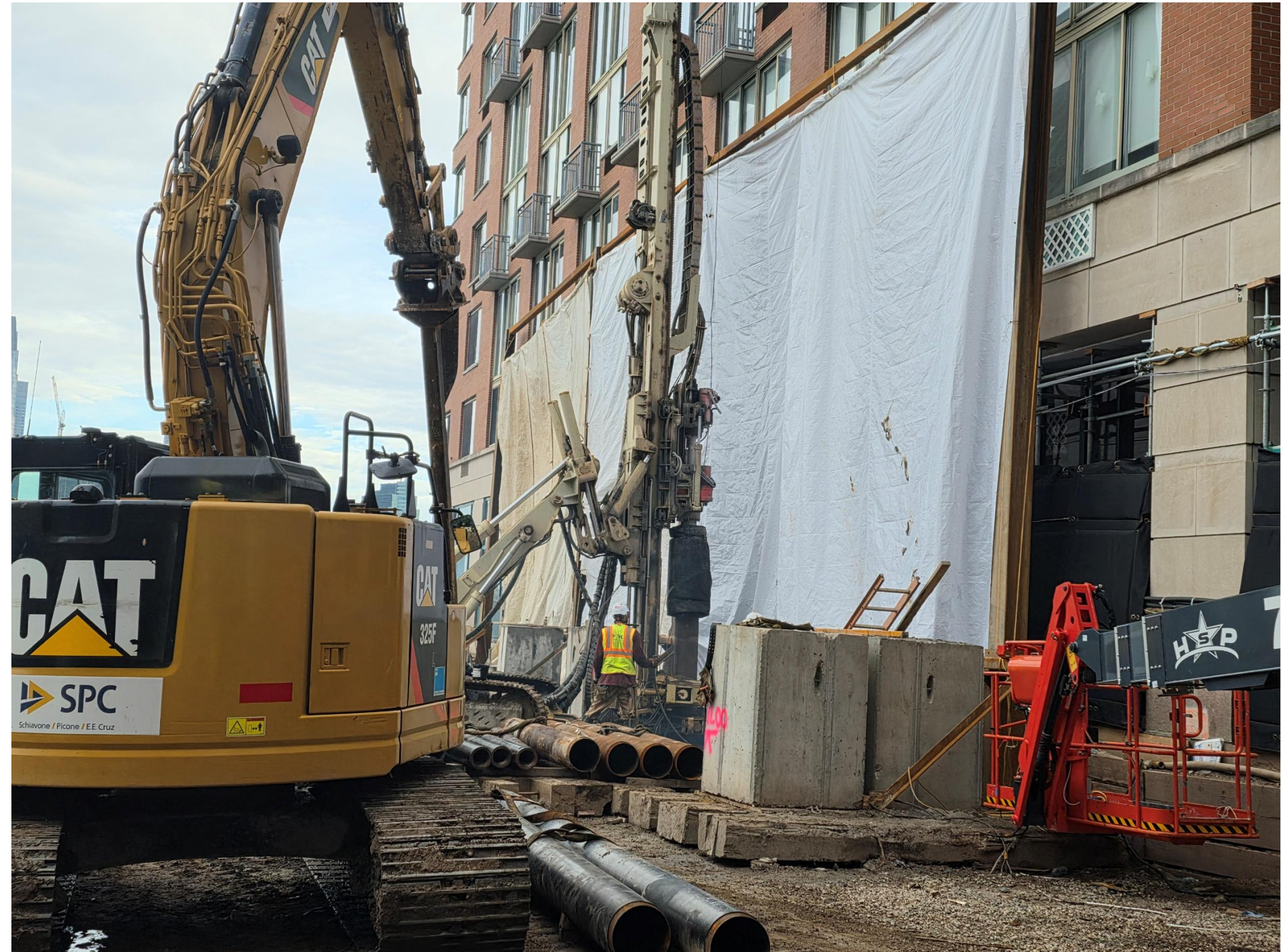
Pile installation along Regatta
