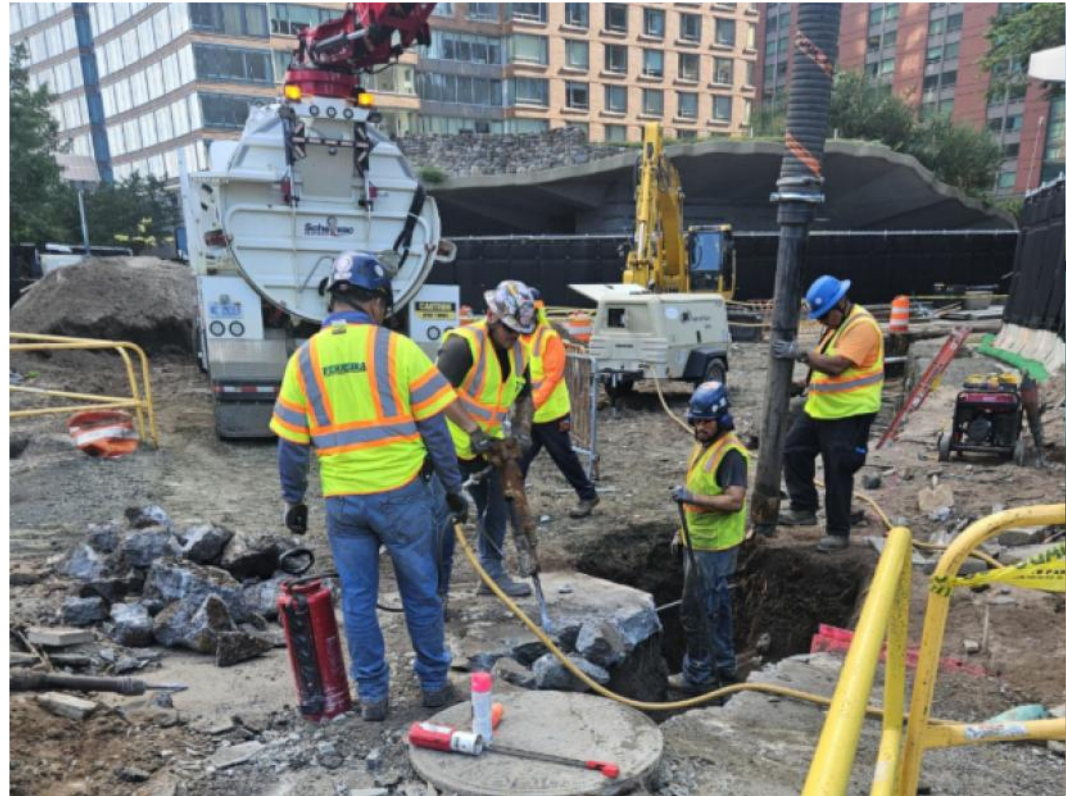
Excavation for electrical ductbank
