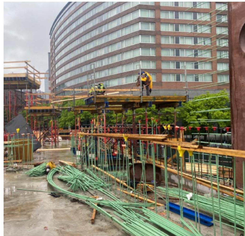
Pavilion concrete work
