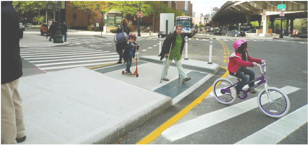
Median Refuge Island
